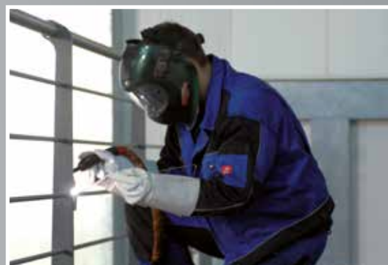
3. TIG welding (DC)*
